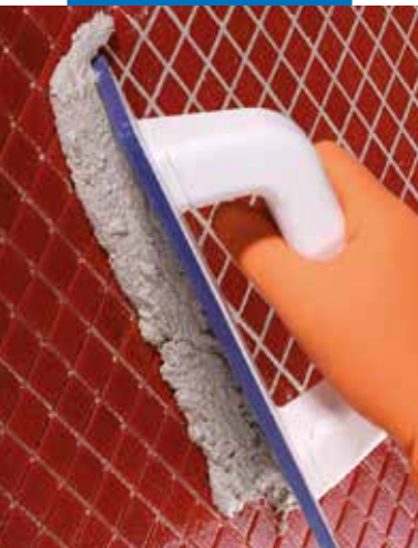
Vtiranje Kerapoxy-ja Design z gumirano lopatico
